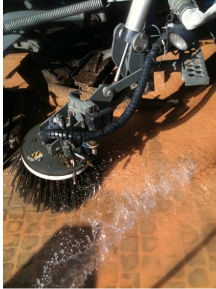
Figure 19: Saturating the pavements while the sweeper truck
