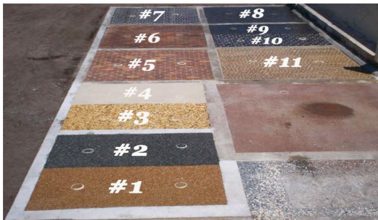
Figure 9: Pavements after completely installed
