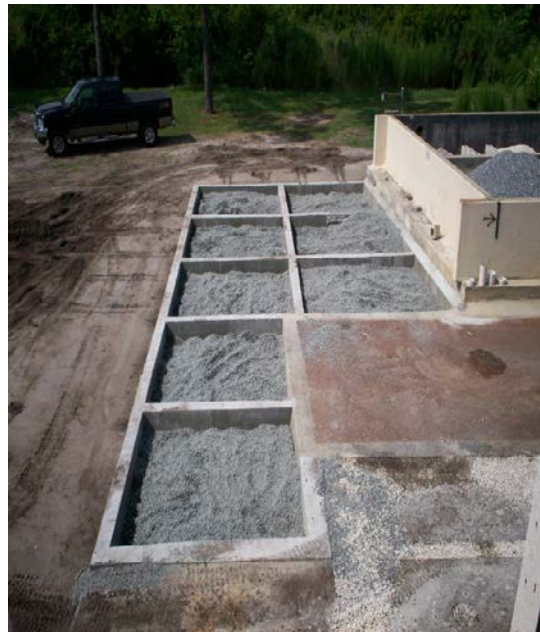
Figure 13: Granite installed over filter fabric prior to compaction
