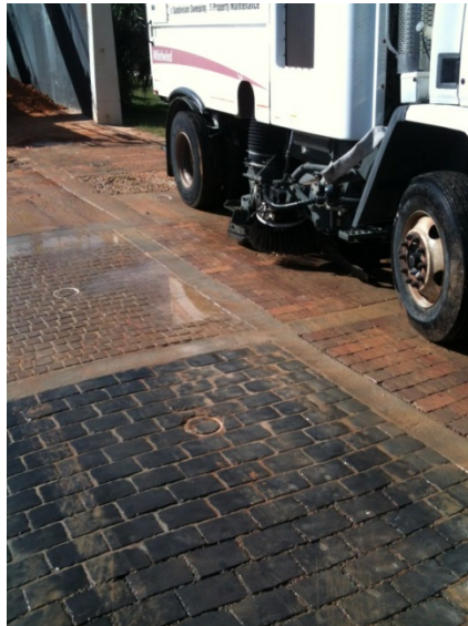
Figure 20: Sweeper truck removing silty-sand soil
