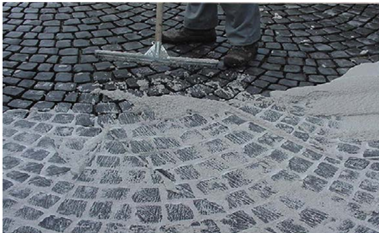
Figure 15: Ecosystems Grout being installed
