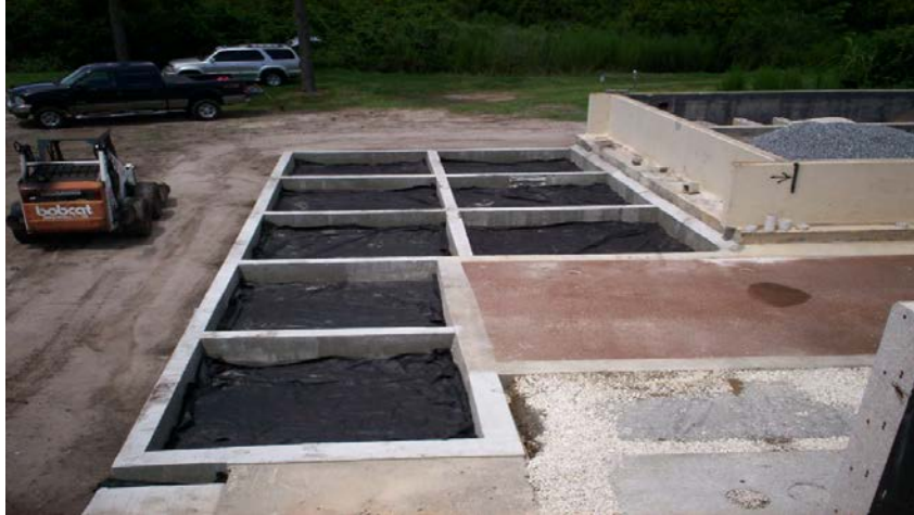
Figure 12: Filter fabric installed
