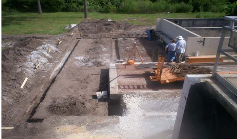
Figure 10: Test area with footings excavated
