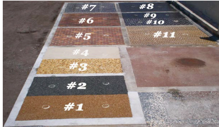
Figure 21: Pavements after completely installed
