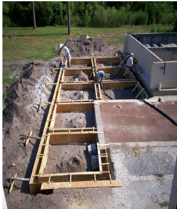
Figure 11: Steel reinforced stem walls being installed
