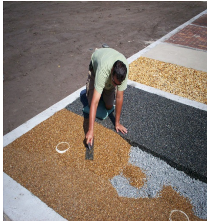
Figure 14: River Rock being installed
