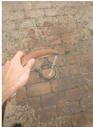
Figure 18: Saturating pavements to optimize soil particle removal
