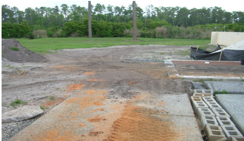
Figure 8: Test area prior to installing pavements
